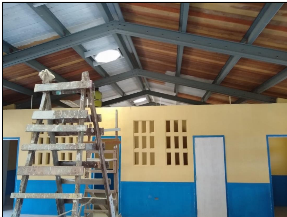
Construction of Good Hope Secondary School - 10 July 2020
