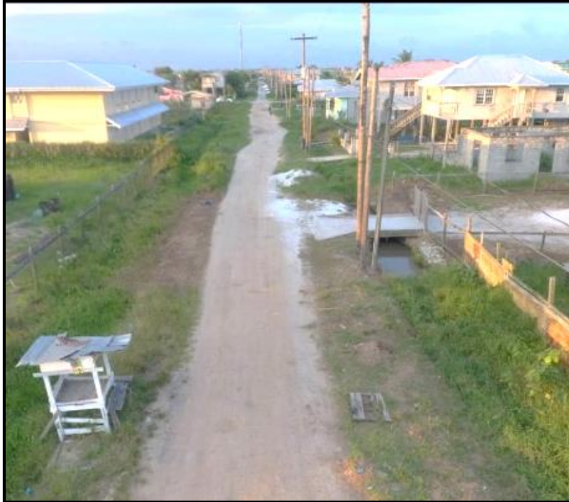
Other road selected instead by the Ministry for rehabilitation under the Contract - 8 October 2020
