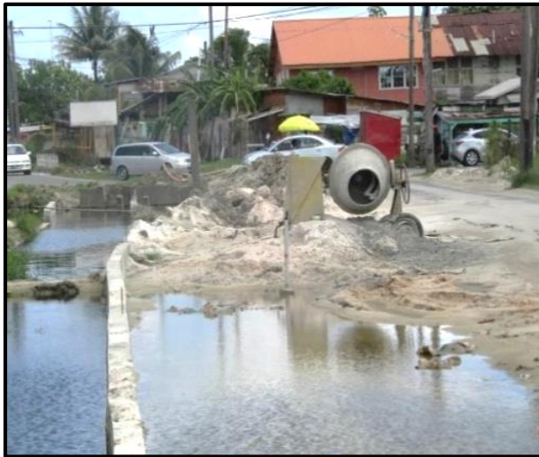
Incomplete works with no road safety and traffic control measures in place on site
