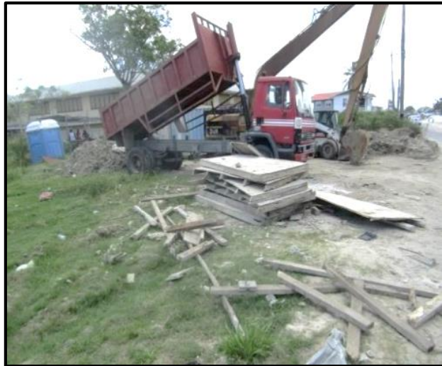
Incomplete works with no road safety and traffic control measures in place on site
