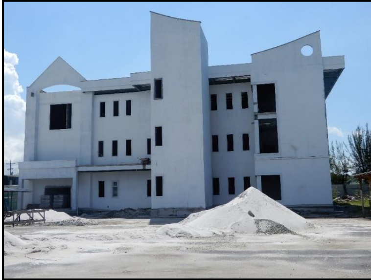
Head Office Building exterior - 8 September 2020
