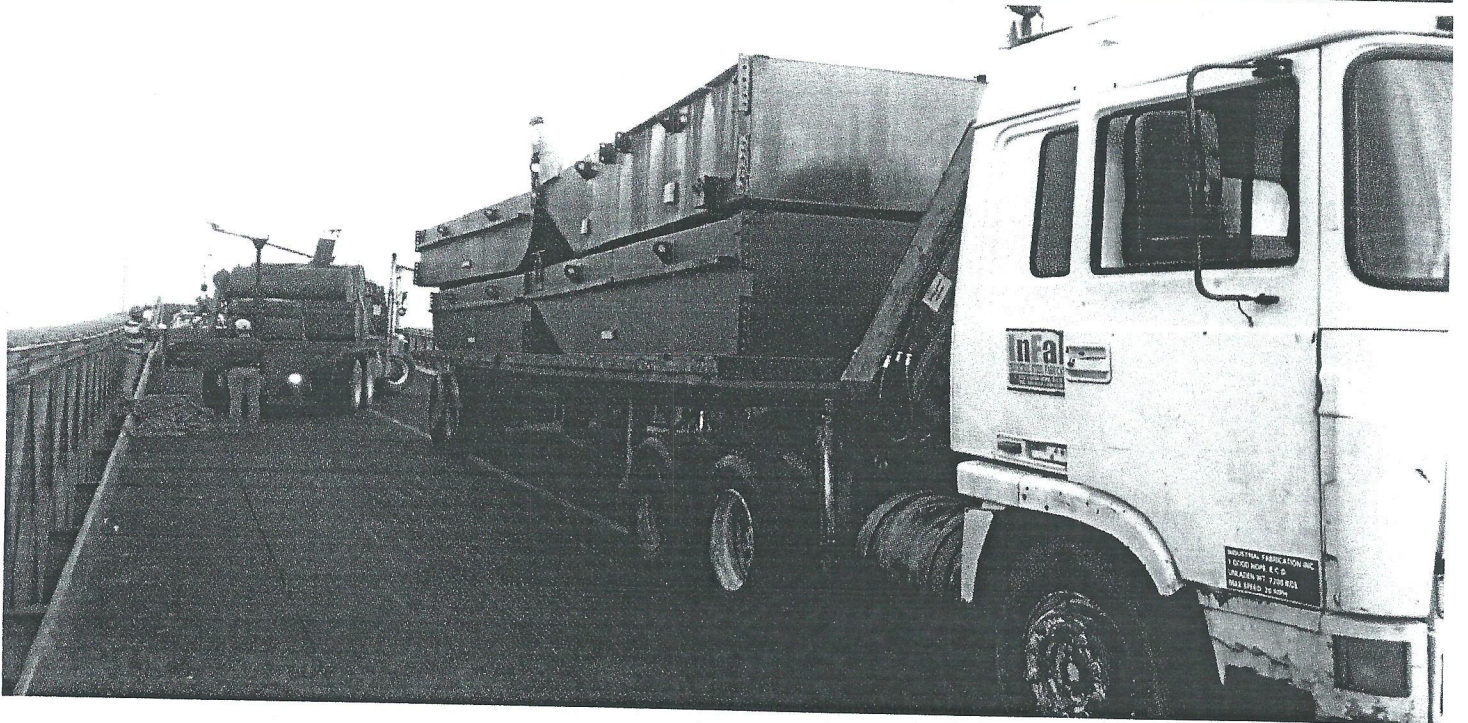
SERVICING OF THE BRIDGE STRUCTURE
